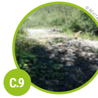
C.9 ALACH-RAUCHWAND A massive stone groyne was shortened by 40 m. → page 12
