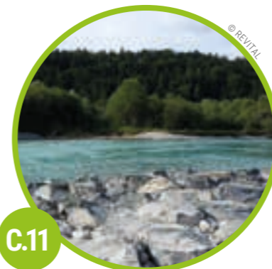
C.11 FEDERAL BORDER TO LECH-SCHLUCHT A stone block spur steers the Lech towards the German side and brings new dynamics to the riparian forest. → page 17
