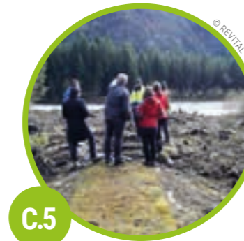
C.5 ELMEN-NUSSAU On the left bank, ten groynes were shortened by up to 70 m. → page 13
