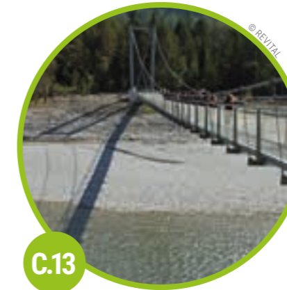
C.13 FORCHACH SUSPENSION BRIDGE The bottleneck is gone! The new bridge is an ideal place for visitors to experience the wild river up close. → page 14
